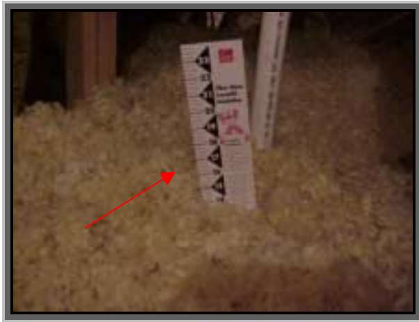
Depth Gauge correctly installed
