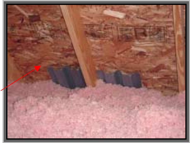
Baffles installed above insulation
